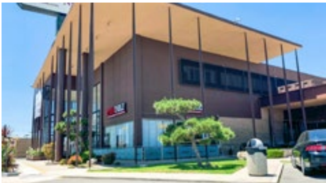
Sumitomo Bank building in Anaheim.
